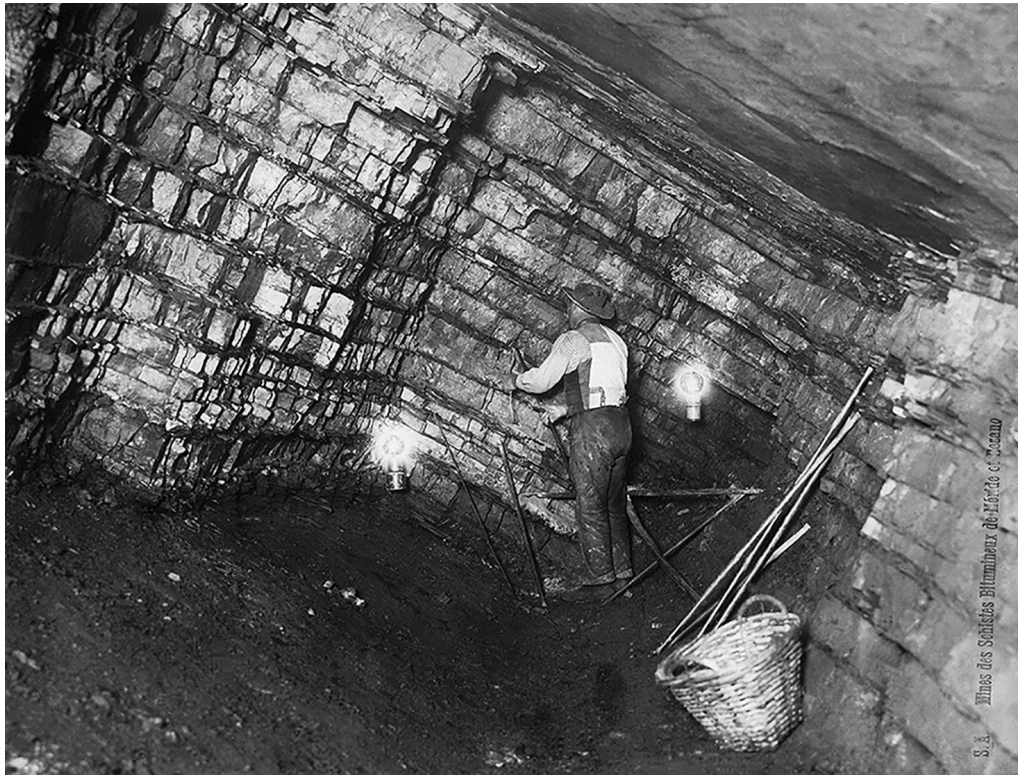
Fig. 2 Miner at work in a tunnel of the mine Cava Tre Fontane near Serpiano at around 1916. © FMSG/archive Sommaruga
